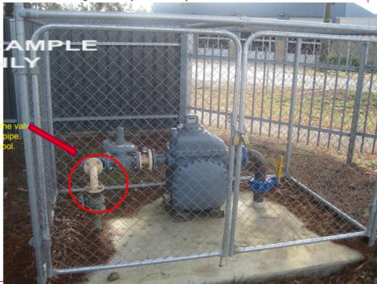
Turn this ball valve 45 degree so the value is at right angle to the gas pipe. This will isolate the gas to the school.
